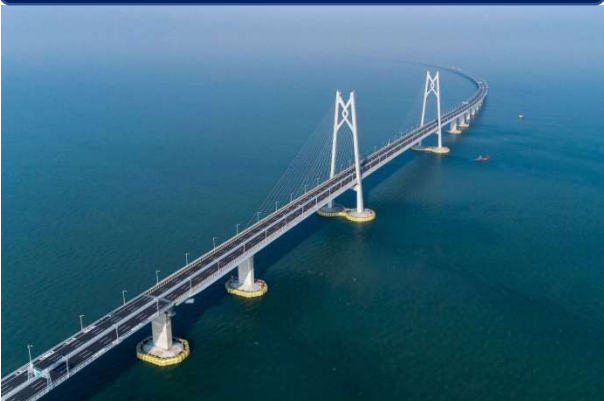
Hong Kong – Zhuhai - Macao Bridge
